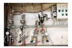
This equipment is used for the automatic switching of ammonia and nitrogen cylinders. When the control verifies that a line is empty, in automatic mode, switching to another line, the switching is notify by an alarm.
